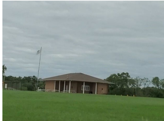
Restrooms (will need additional)
